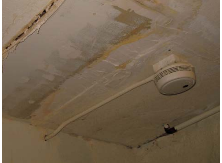
Collapsing ceiling from mold and water damage
